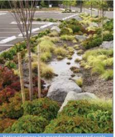
Native plantings in a meandering vegetated swale could function as an urban stream to manage stormwater and treat roadway runoff
